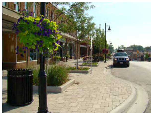
Curb bump out defines on street parking areas and provides traffic calming while landscaping elements animate the pedestrian zone
