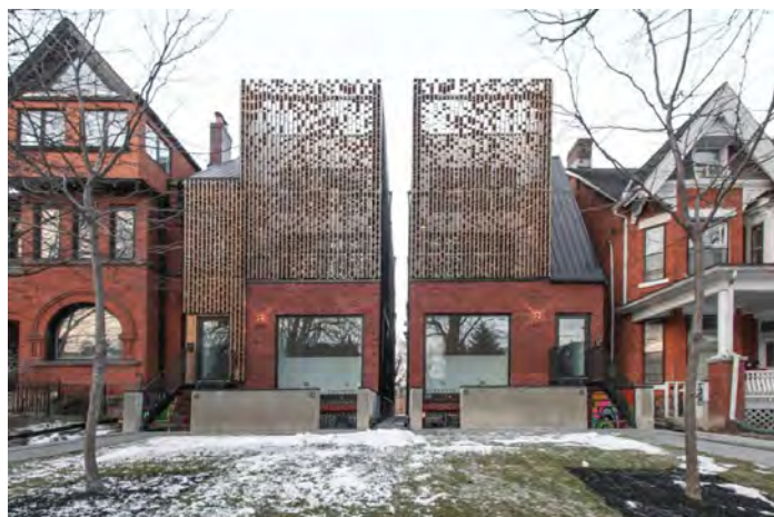
Consistent ground floor height and materials
